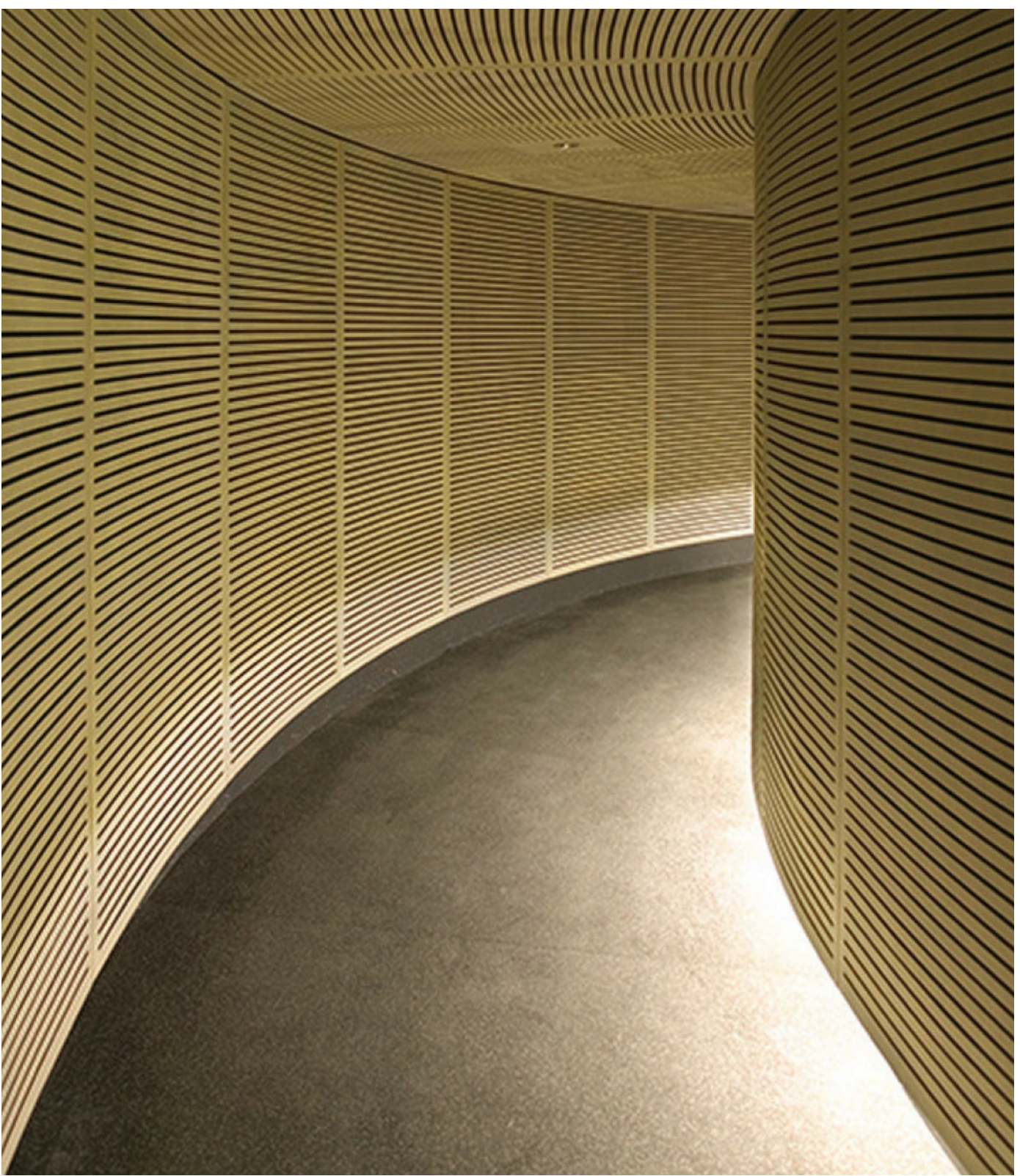
Figure 3.48 Linear luminaires floor washing behind a skirting board, Eden Project Visitor Centre. (Arch: Grimshaw Architects; Lighting: Mindseye; Photo: Adam Parker)
