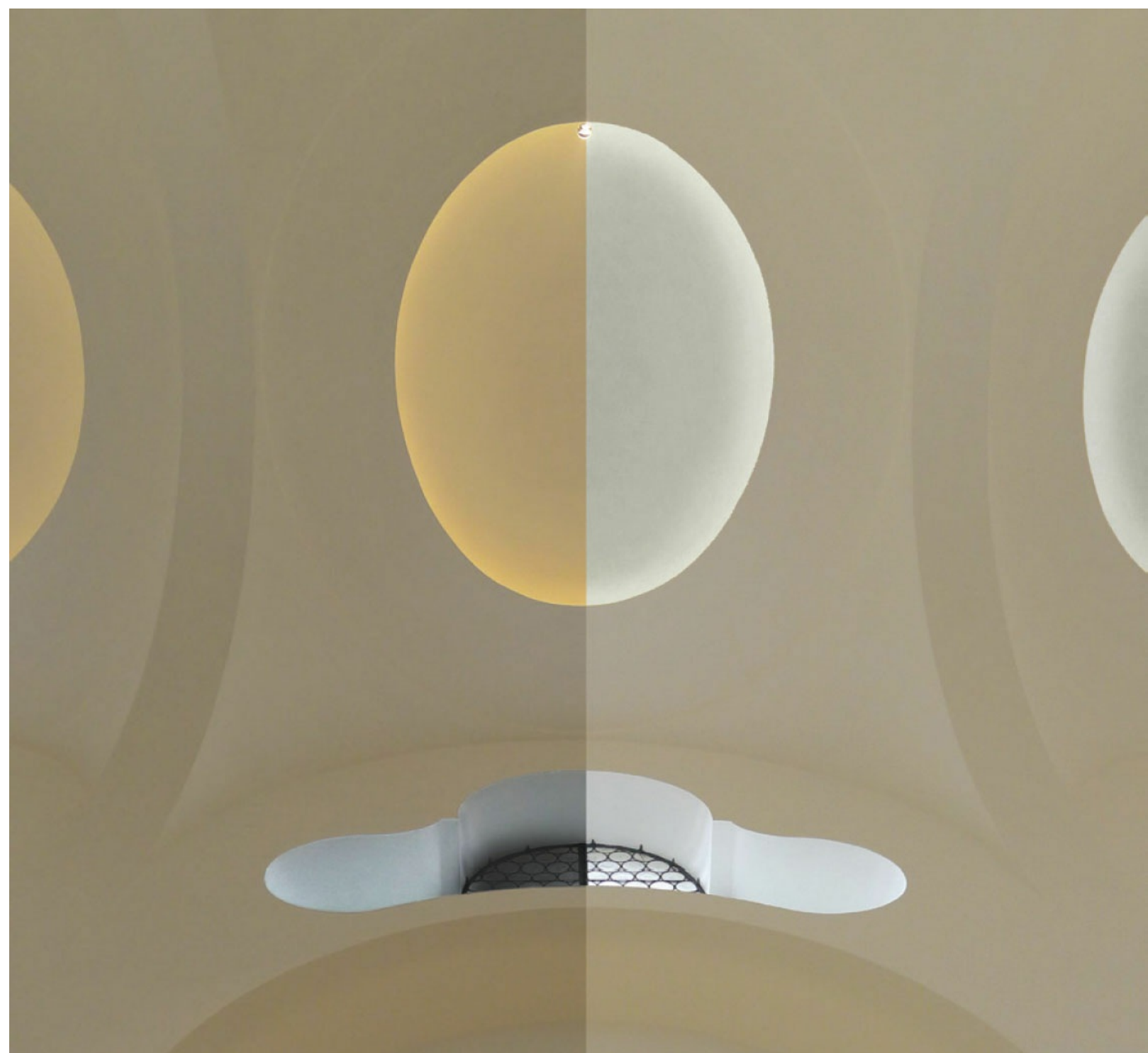
Figure 4.32 Colour temperature of the light within the building changes from 2700K in the morning to 4000 during midday returning to 2700K in the evening St. Moritz Church, Augsburg.
