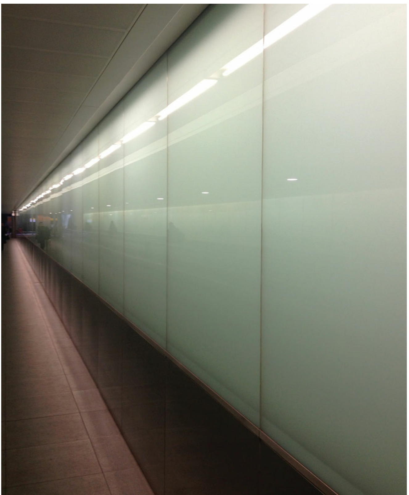
Figure 6.01 An example of luminaires unintentionally reflected off glass panels.
