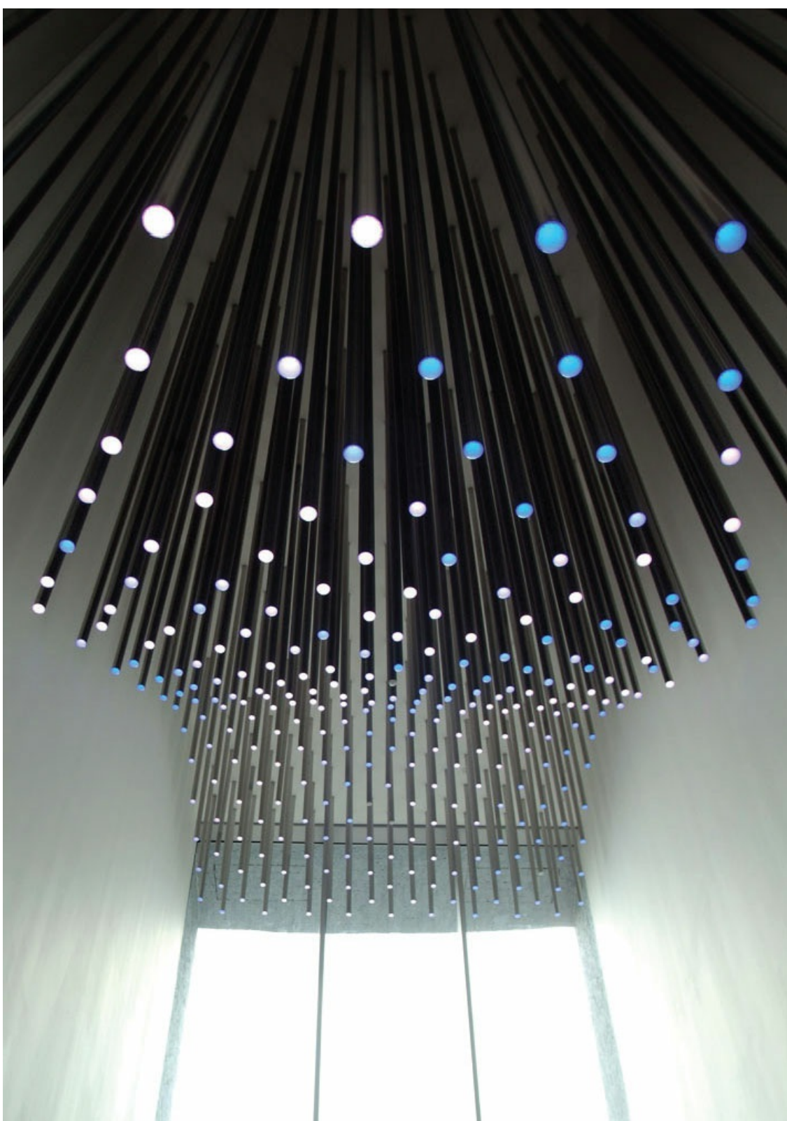
Figure 2.17 Bespoke LED tube using recessed light from the shelf lenses. (Mindseye Lighting)
