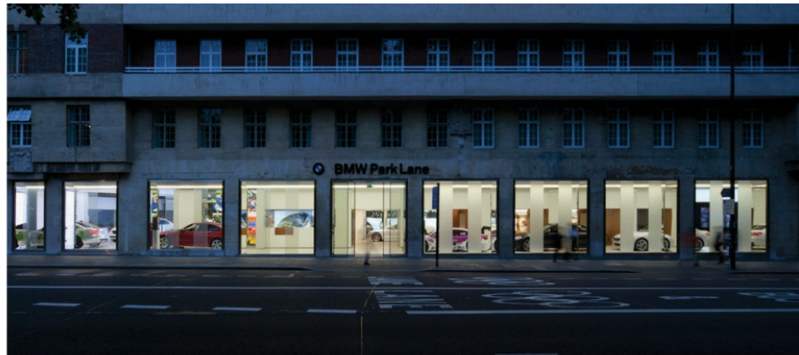
Figure 6.36 Most verticals are treated showing that BMW Park Lane is 'open for business'.
