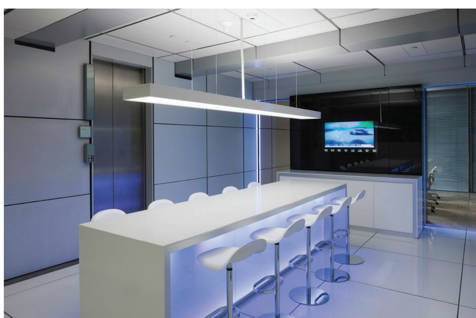
Figure 2.38 Bespoke pendant with up- and down-lights on separate circuits. (HSBC, Hong Kong)
