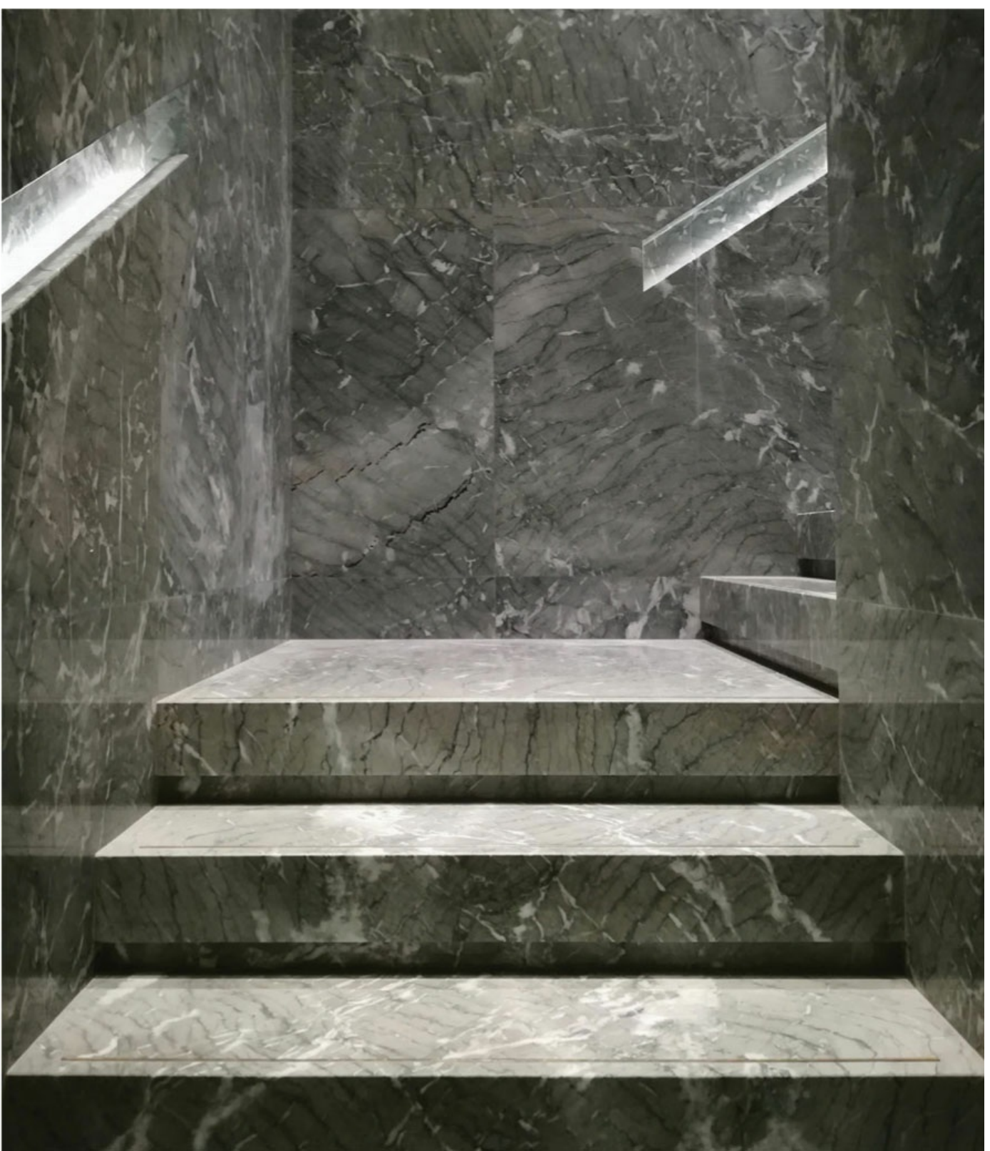
Figure 6.11 Handrail lighting not visible-the reflective marble made it difficult to hide the integral linear luminaire. (Photo: Antoine Huot)
